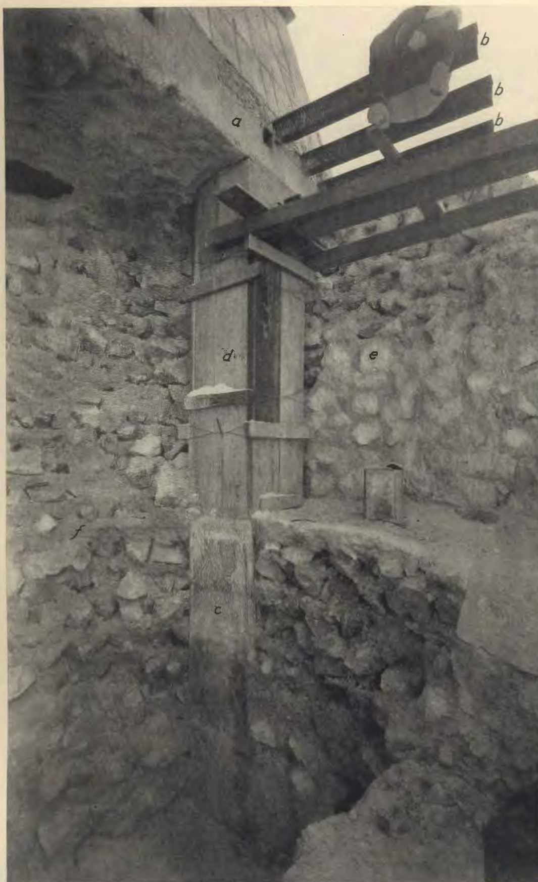
CONCRETE COLUMN CAST ON TOP OF COLUMN 5, TEMPLE OF THE CHAC MOOL
