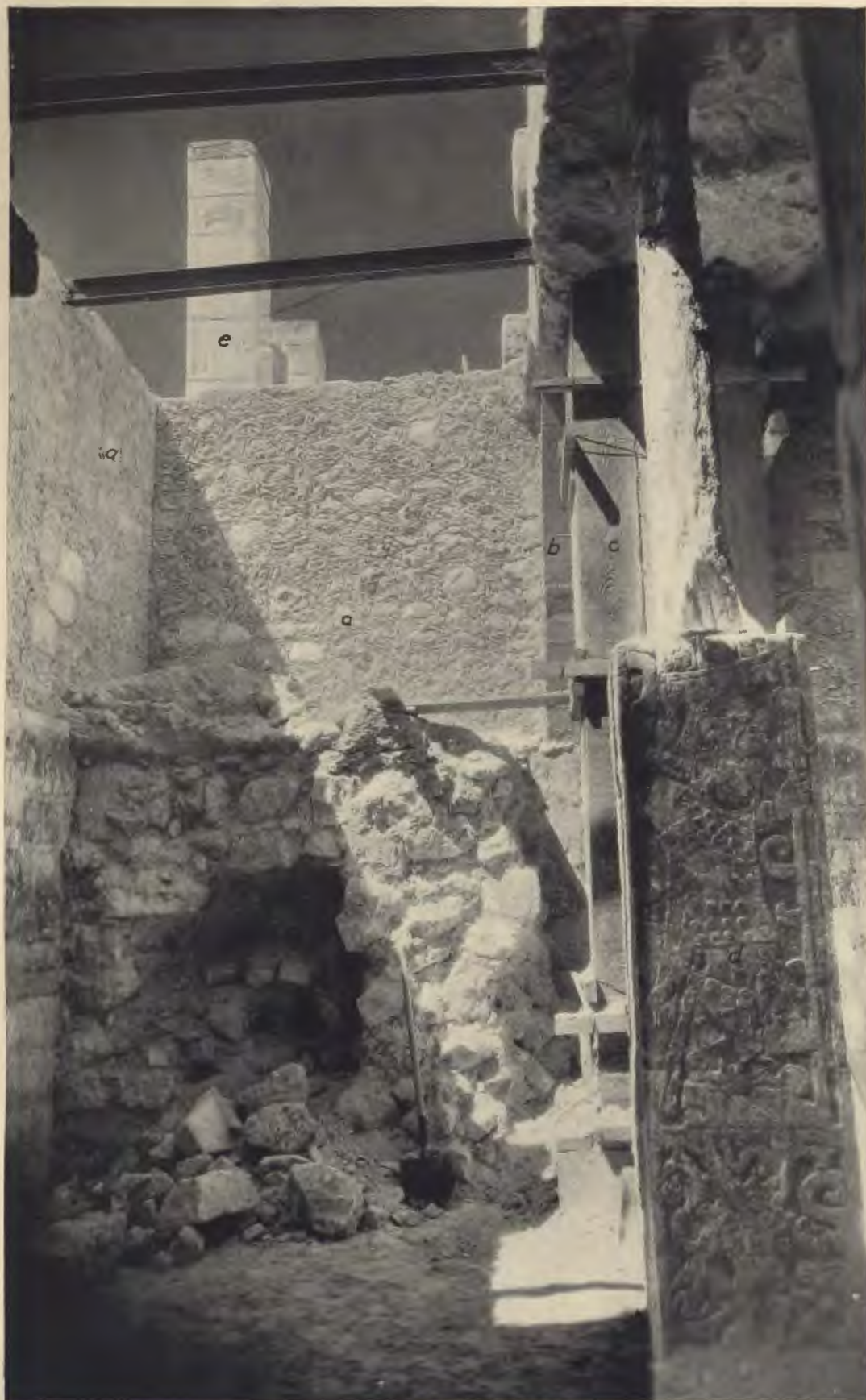
SOUTHEAST CORNER, TEMPLE OF THE CHAC MOOL, SHOWING LAST INCREMENT OF ORIGINAL FILL
